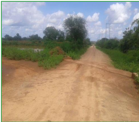
Road Run-off harvesting through cross culvert to a farm pond.
