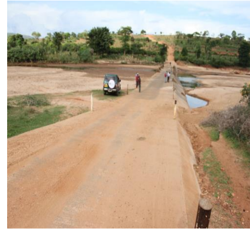
Non-vented road crossing/Drift which provides crossing and sand storage.
