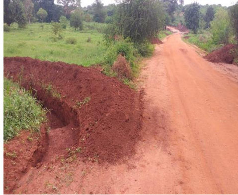
Green Road with miter drains to nearby farms.
