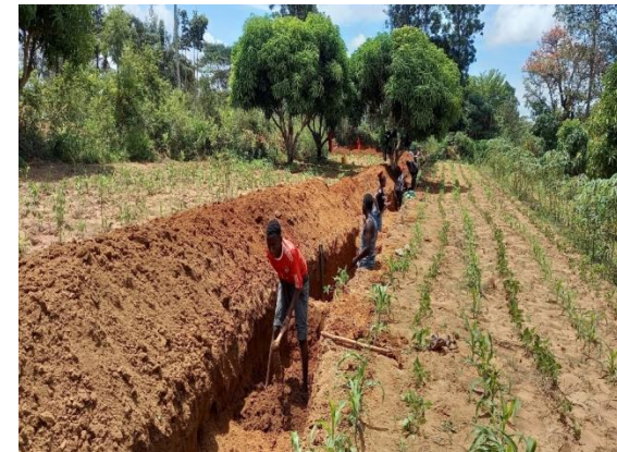
Excavation of Road side mitre drains for road runoff harvesting.
