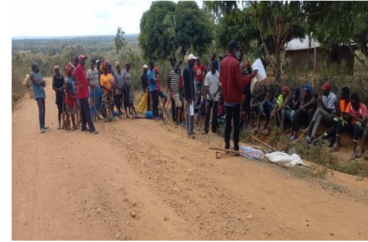
Community empowerment program for excavation of roadside mitre drains.
